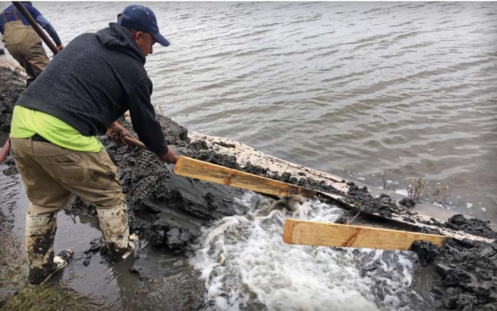
Once filled, the SOX system was shaped to integrate naturally into the existing shoreline. The SOLitude team made additional considerations to extend the length of key pipes and drains located within the bank. The restoration work was completed with the installation of native plant species in the precious littoral zones along with sod, which were planted to give the lake a [living shoreline](#) and help filter excess nutrients from entering the
