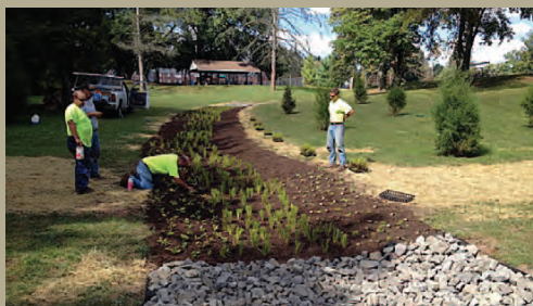
Fall 2013 - Installation of 2-inch plugs according to planting concept plan. Installation labor provided by township staff, project oversight provided by SOLitude
