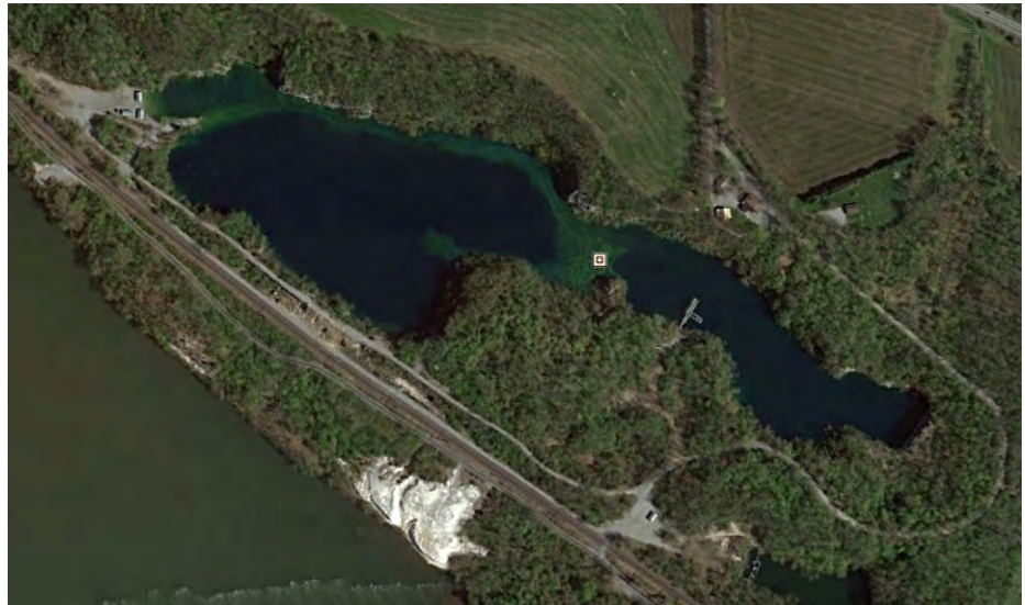
Figure 1. Aerial view of Billmeyer Quarry, with the Susquehanna River to the southwest. The west basin (left) is the larger and deeper of the two (photo from Google Earth).
